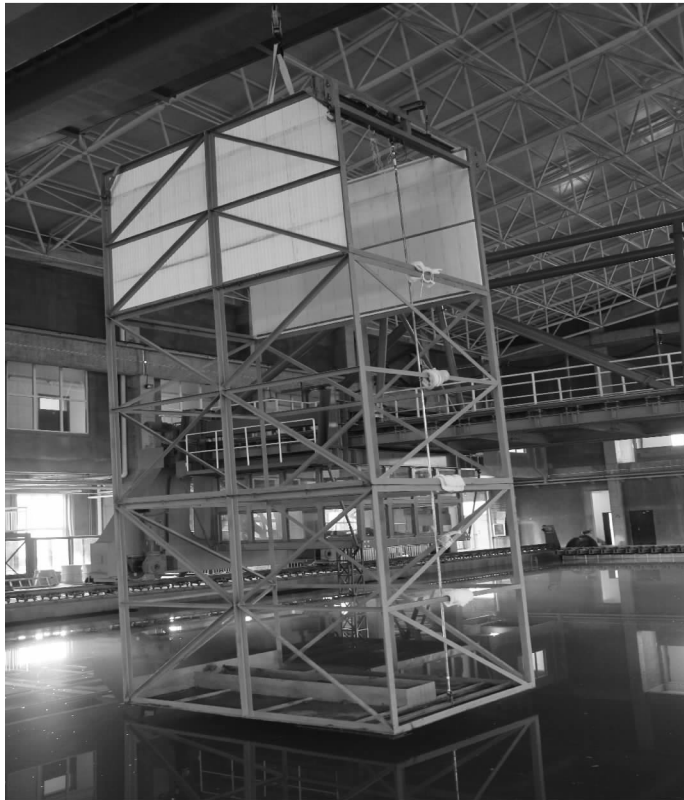
(a) 吊装 (a) Lifting
